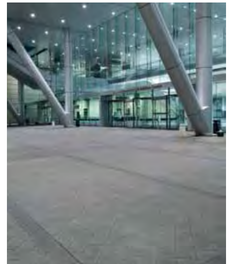
Above and Left Photos: Boston Convention Center, South Boston, MA; Landscape Architect: Richard Burck Associates, Somerville, MA; Size & Color: 8" x 8", A80014, #A80016; Finish: Ground/Tudor®
